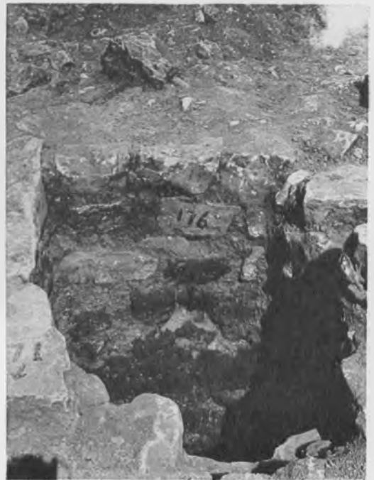
4. MASONRY IN NECK OF, CISTERN 176
