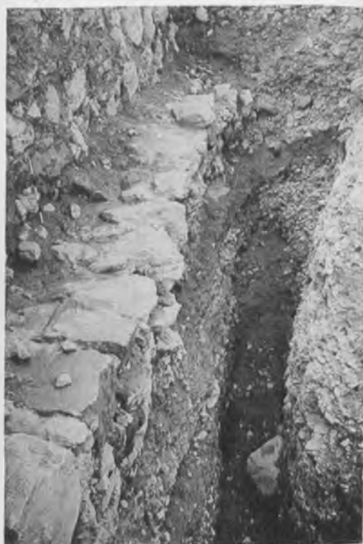
4. INTERIOR OF EAST WALL SHOWING SHELF MADE BY WIDE FOUNDATION
