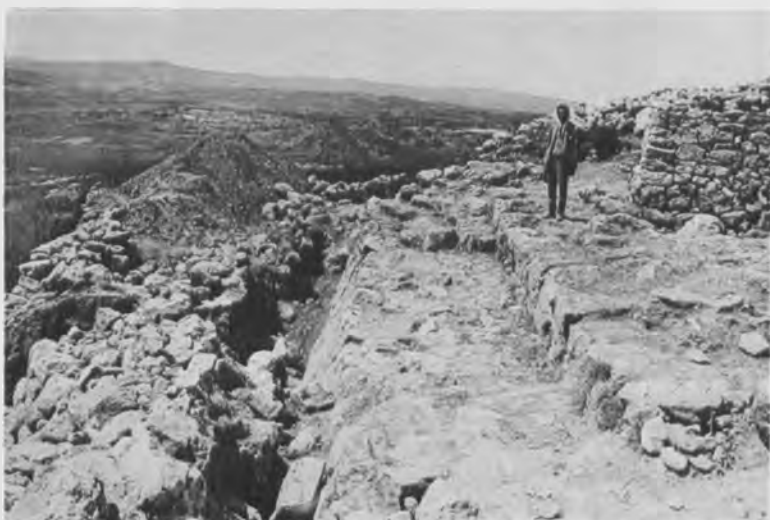
3. EXTERIOR OF WALL WITH REVETMENT BUILT AGAINST IT
