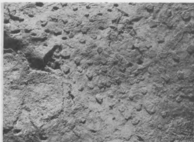
1. DETAIL FROM WALL OF CISTERN 33 SHOWING HOW PLASTER WAS KEYED TO WALL
