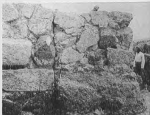
7. JOINT BETWEEN JAMB AND BLOCKAGE, NO. 6
